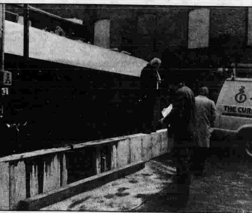
FUEL SPILL — Two hundred gallons of fuel accidentally overflowed a 10,000-gallon fuel tank this morning in back of the Thrall building, 5 Glen Road, Manchester. Here, Manchester Fire Capt. Rudy Kisman stands on top of a cement retainer surrounding the tank, which trapped the spill until it was cleaned up.
